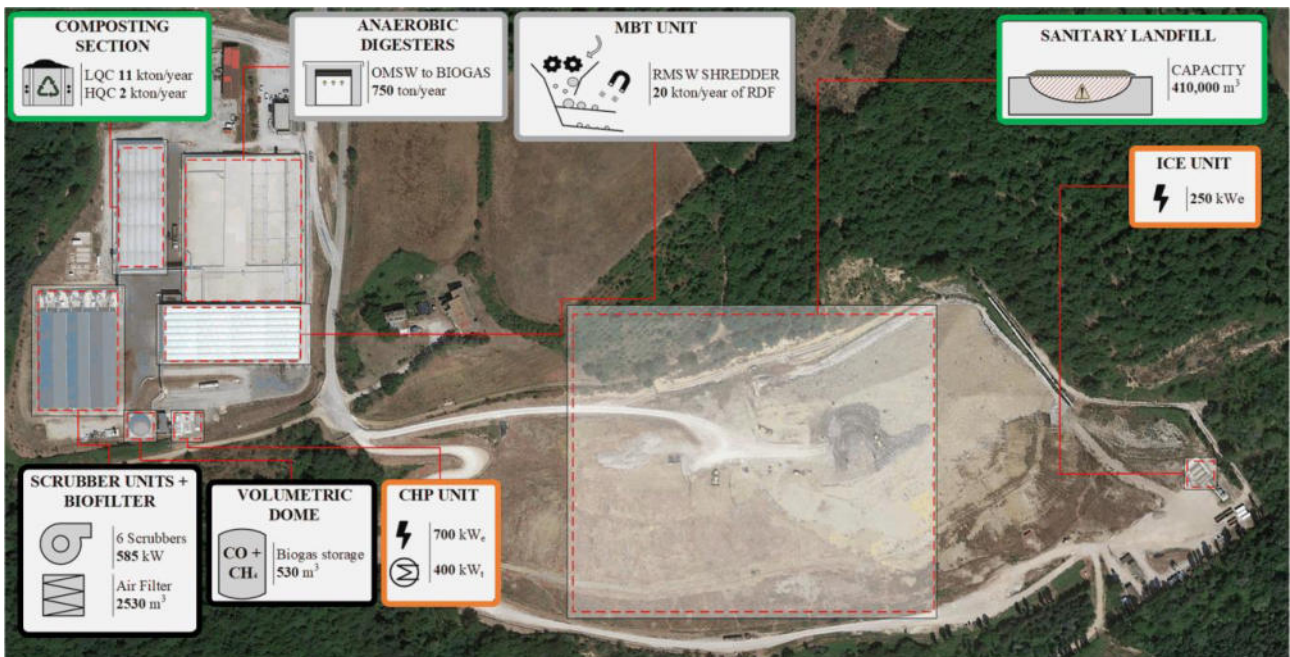
Fig. 2-1. Overview of the waste treatment facility under analysis, with detailed infographics of the relevant sections.
